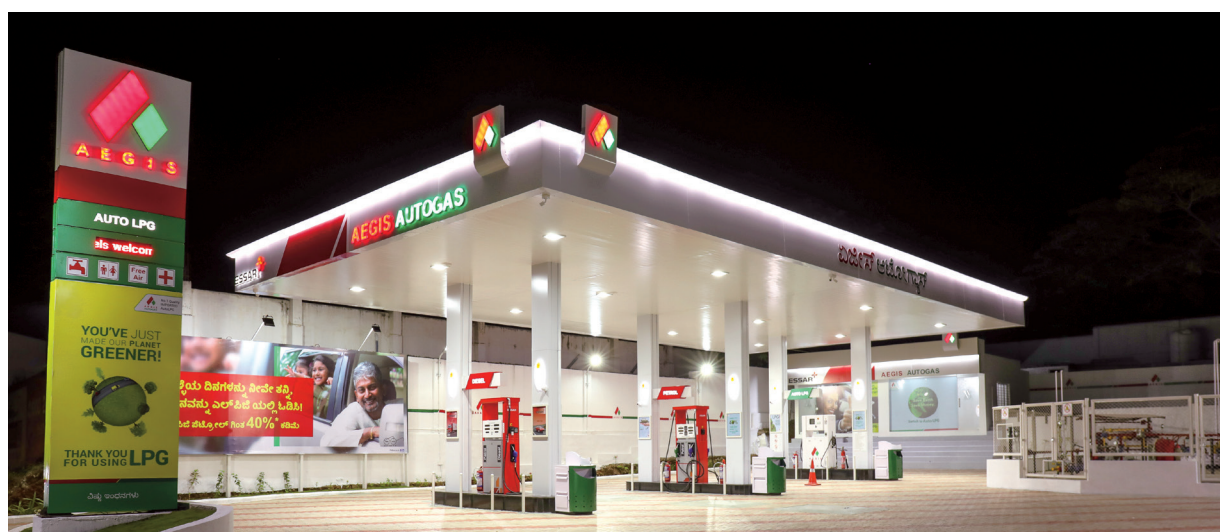
Newly commissioned multi-fuel station
